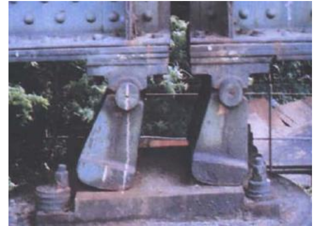
Fonte: BRIDGE INSPECTION MANUAL – NY'S DOT
