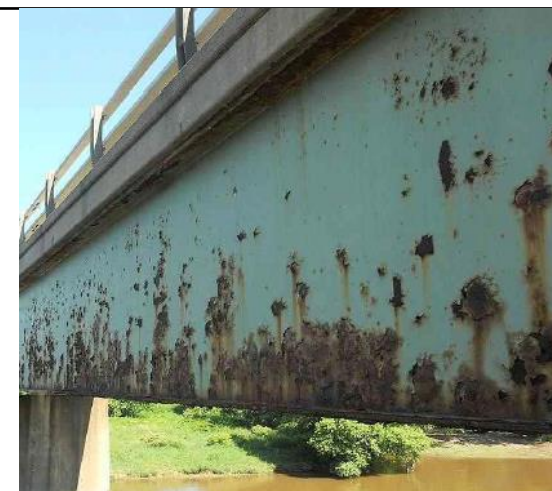
Fonte: BRIDGE INSPECTION MANUAL – NY'S DOT
