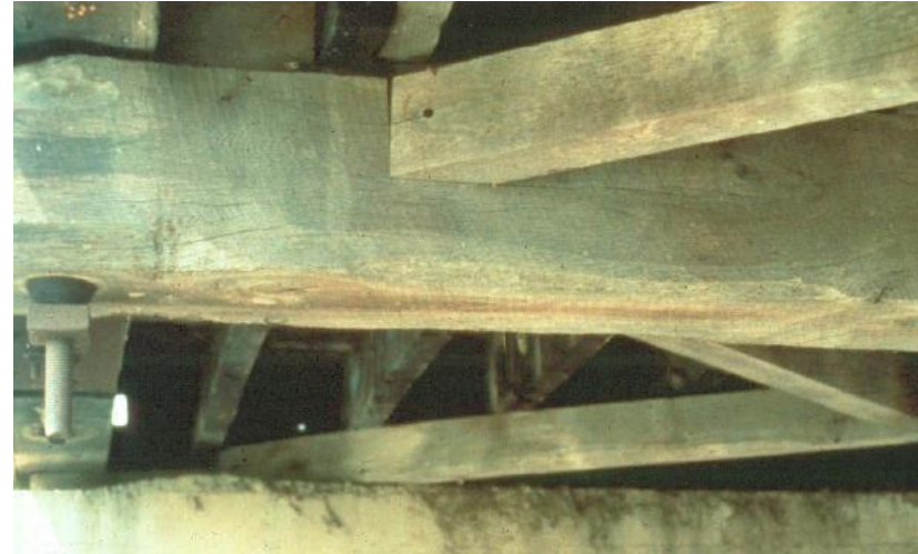
Fonte: BRIDGE INSPECTION MANUAL – NY'S DOT
